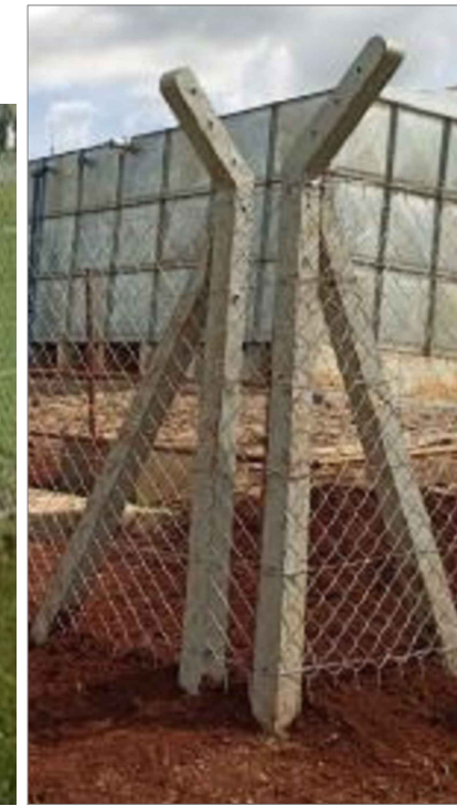
Image of Corner Post Type 1 for corner angle < 135°
