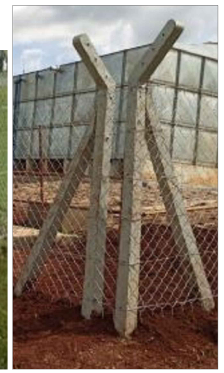
Image of Corner Post Type 1 for corner angle < 135°
