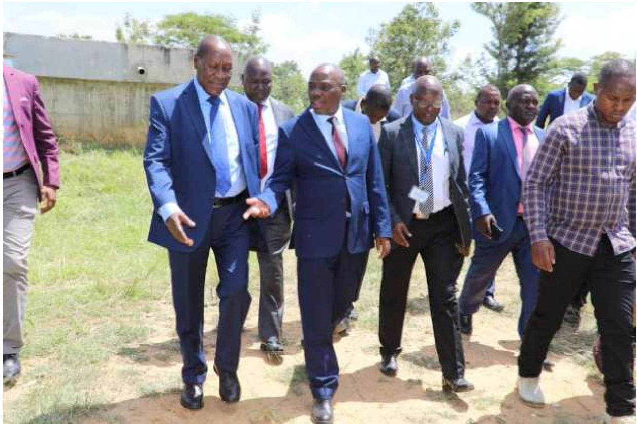
TAW/WDA CEO, Eng Fredrick Mwamati takes the PS Dr. Paul Kiprono Rono and Kitui Governor H.E Dr. Julius Malombe to Kwa-Ngindu Tank. This is a component of Masinga-Kitui Water and Sewerage Project with a capacity of 15000m 3
